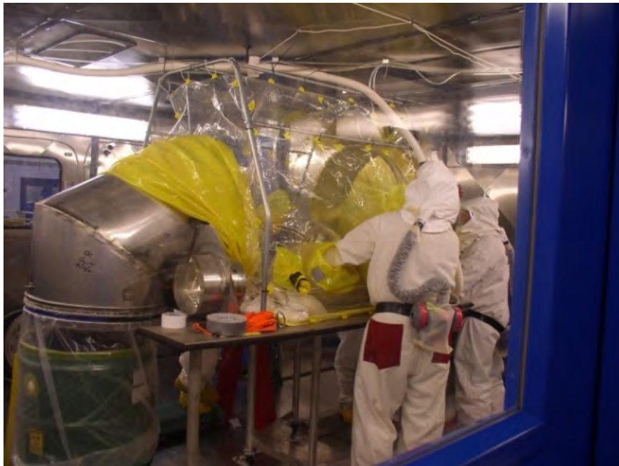
Performing repack operations in a permacon in T-Plant canyon.
